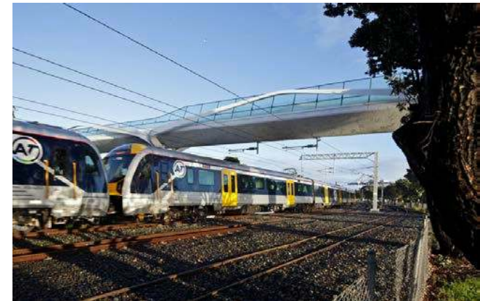
Bridge barrier example from New Zealand
