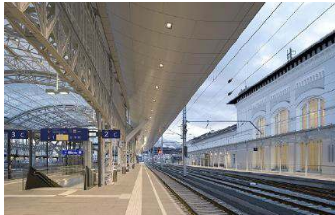
OCS at station example Salzburg, Austria
